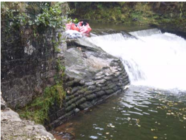
Phase 1 site preparation
