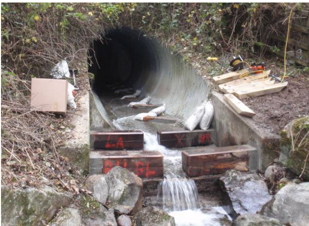
Technical easement "in progress" on the confluence of the Pont Bren
