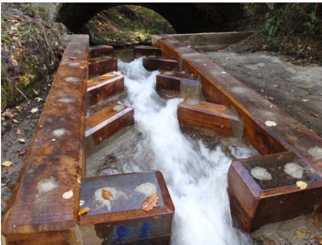
Technical easement on the confluence of the Pont Flocksman
